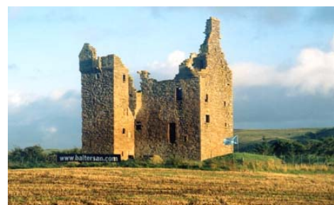
Baltersan Castle (before restoration!) viewed from the north west.
